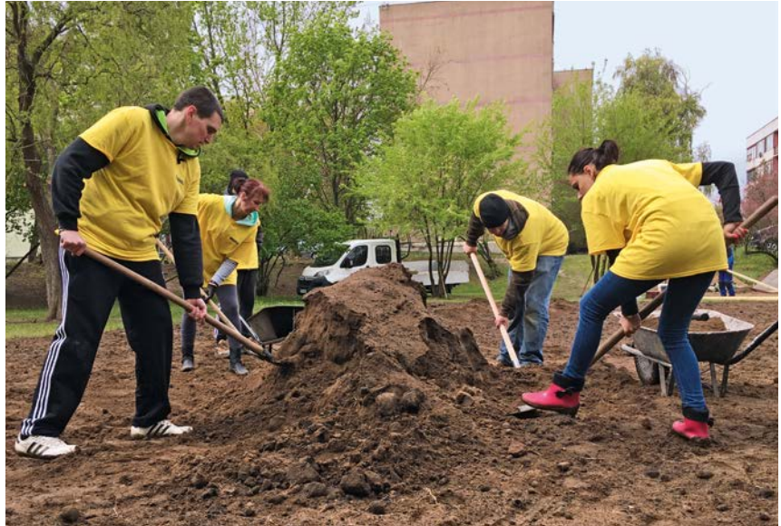
Employees from our location in Balassagyarmat/Hungary help to construct a playground for local children.
