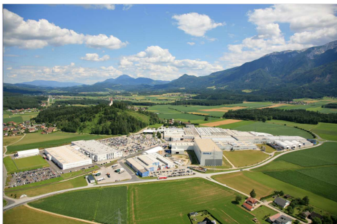
All MAHLE plants in Austria, like this filter plant in St. Michael/Carinthia, obtain their electricity from hydropower and other renewable energy sources.
